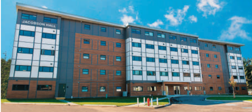
In 2018, Triple M Housing and Metric Modular broke through an industry barrier when they constructed the tallest wood framed modular housing structure in Canada. Jacobson Hall at Trinity Western University won first place from the Modular Building Institute, an organization that represents modular builders from 25 countries.
